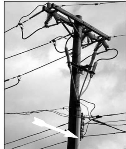
Photo #1--Riser pole is supplying high-voltage lines (arrow).
