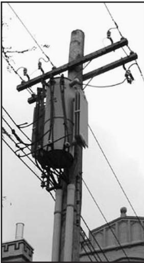
Photo #3--4kV transformer supplying secondary risers.
