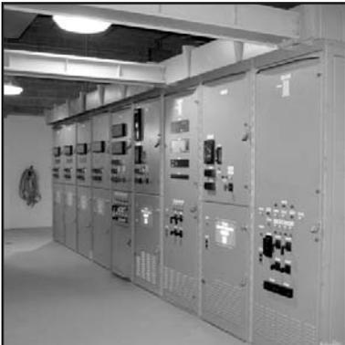
Photo #4--Circuit breakers are housed in locked cubicles to eliminate the chance of anyone casually entering these areas.
