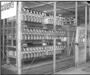
Photo #3--Capacitor banks reside in cages that provide a buffer zone between you and the exposed electrical conductors.
