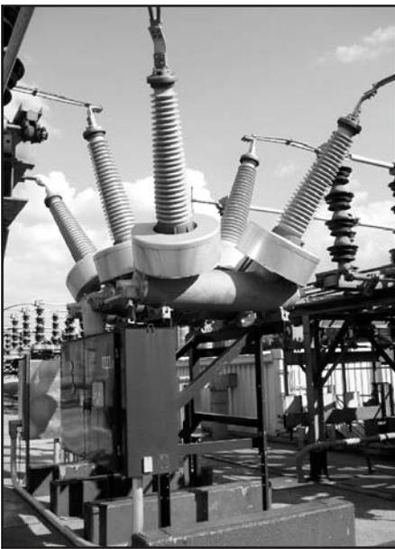
Photo #12--Sulfur hexafluoride gas is used to insulate and extinguish arcs in electrical components, such as circuit breakers.
