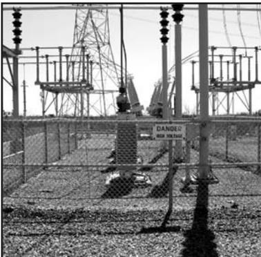
Photo #5--Lightning arrestors are found behind fences. Remaining outside of these fenced areas ensures your safety.
