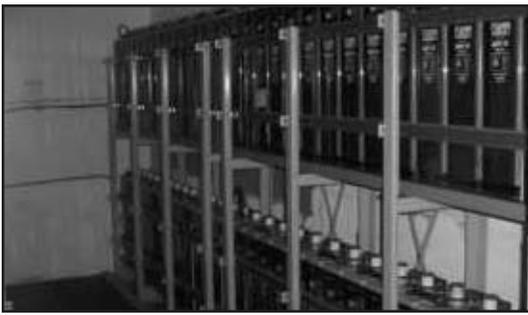
Photo #11--Each substation has two battery rooms, with each room holding 30 to 40 car-type batteries.
